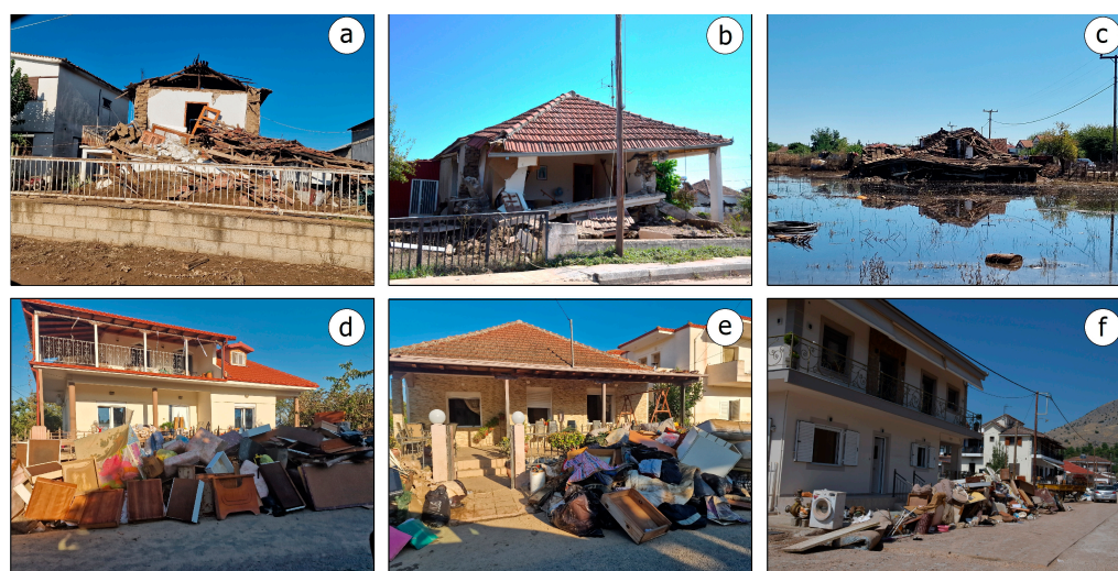
Figure 5. One of the main risks that emerged from flood water in the affected areas is related to flood waste management. Many masonry buildings suffered collapse (a–c), increasing the final flood waste volume. Many villages of the Thessalian Plain were inundated by flood water, resulting in the destruction of household equipment (d–f), buildings, and facilities. The resulting piles comprised hazardous materials with a high potential to affect not only the environment but also public health. Their collection, treatment, and disposal were a challenge for the authorities managing the disaster impact.
