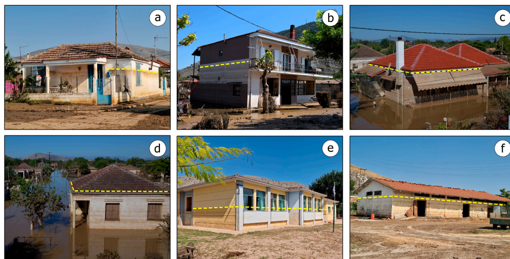
Figure 4. Typical views of structures in the flooded Thessalian Plain including (a–d) houses, (e) schools, and (f) warehouses. The level of the flood water has been imprinted on the walls and even on the roofs after receding and it is highlighted in the photos with a yellow dotted line. The flood water in many cases inundated not only the ground floor, but also the first floor of many houses, threatening residents and causing the total destruction of household equipment.
